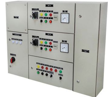
Control panel - form 3b
