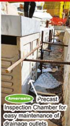
Amerasia Precast Inspection Chamber with access cover for maintenance of drainage outlets
