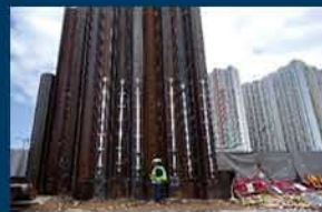
Piling Magnetic Tuned Mass Damper
