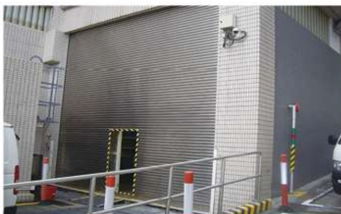
Stainless Steel Shutter at CLP's Station at Tsz Wan Shan Office
