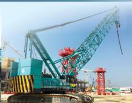
KOBELCO 7250S 履帶式固定吊臂：61m
